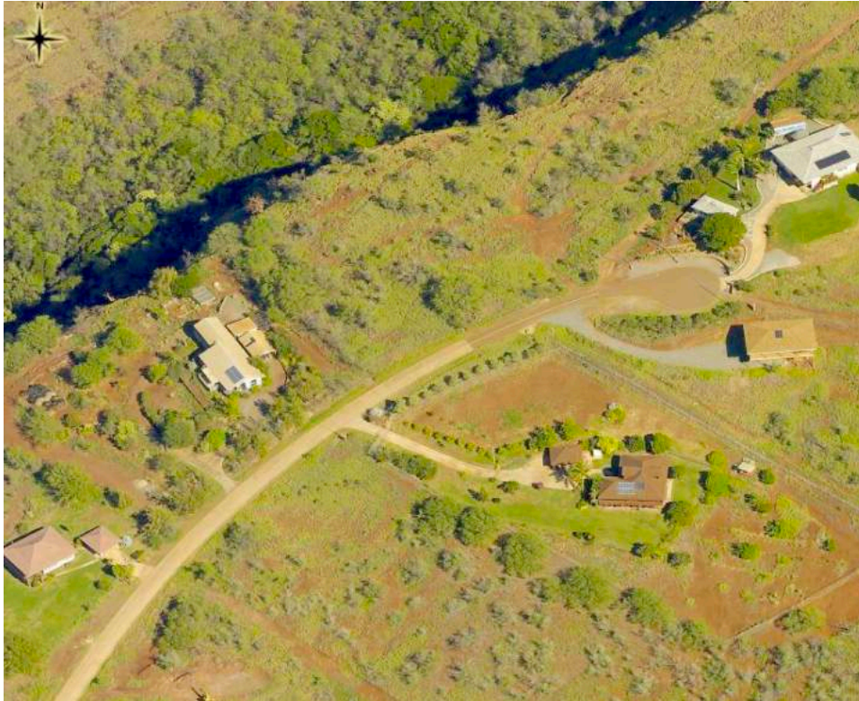
South view of Lot 30. Lot centered between homes and gulch.
