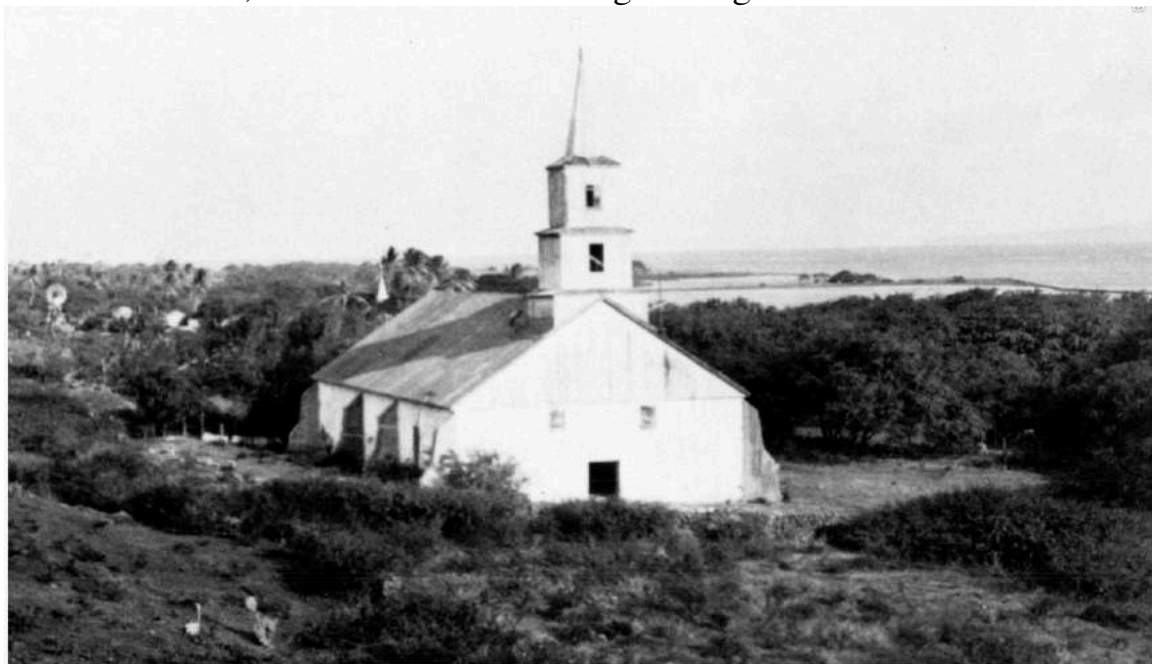
First church on Molokai built by Protestant missionaries in 1844 in Kaluaaha when it was Molokai's first and principal town. Lacking a harbor, it was eventually surpassed and supplanted by Pukoo and Kamalo, and both of them eventually by Kaunakakai as the irrigated plains of the saddle lands
