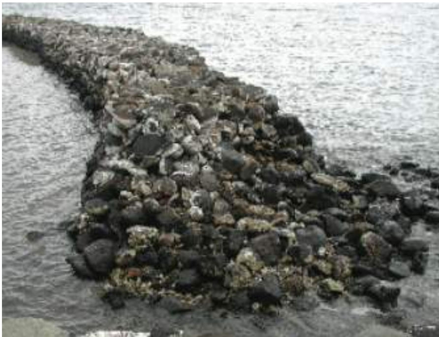
Above: Collapsed Kahinapohaku fishpond wall before reconstruction showing interior rock wall construction.
