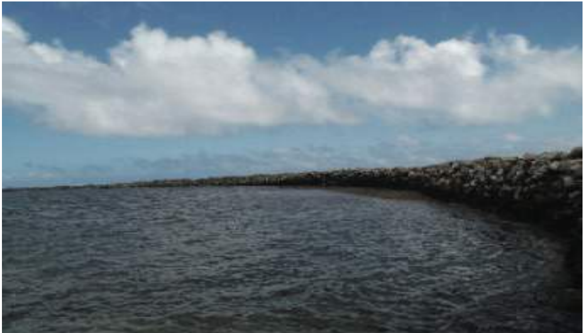
Above: Kahinapohaku fishpond rock wall after rebuild.
