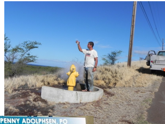
Mervin Dudoit, checking the cleanliness of water during flushing the distribution system
