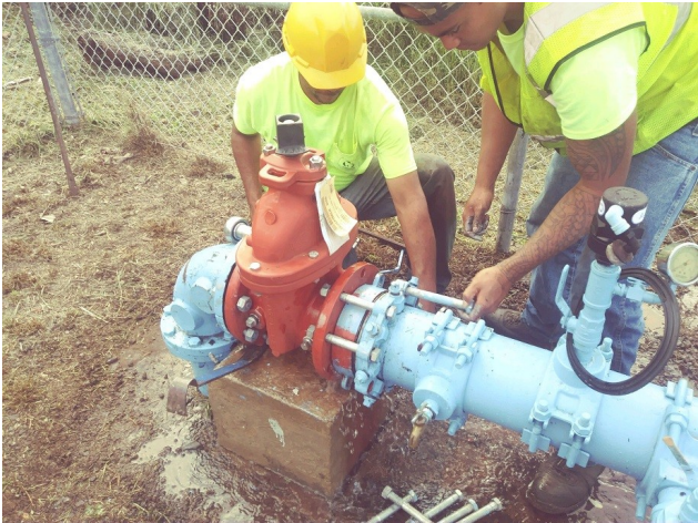
John Colon (Koa) and Anoi Lima English working to replace the gate valve at the pressure reducing site.
