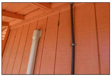
**Evaluation:** No wood rot or Termite damage observed. Siding is in fair intact condition, and paint is in fair to poor faded
