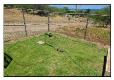
**Evaluation:** Standard 7 Ft tall galvanized fencing supported by tubular framework. Most sections undamaged and secure. Hinged gates function and most are in alignment. Generally in fair condition, aging extended due to dry climate. Expect to repair as needed under the Operating Budget, not Reserves.
