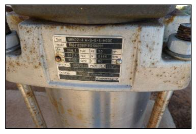
**Evaluation:** Replaced 15 HP Grundfos "cam" pump in 2015. Expect eventual replacement of pump, flow meter and gate valve on this cycle.
