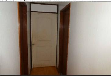
**Evaluation:** Doors are aged and in fair to poor condition. Recommend partial replacement of 2 doors on this cycle.
