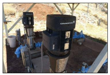
**Evaluation:** Replaced 15 HP Grundfos "cam" pump in 2015. Expect eventual replacement of pump, flow meter and gate valve on this cycle. Coordinate with Booster Pump #1 Replacement. Both boosters pump from DT 100,000 USG tank #1 to DT 150,000 USG tank #2.
