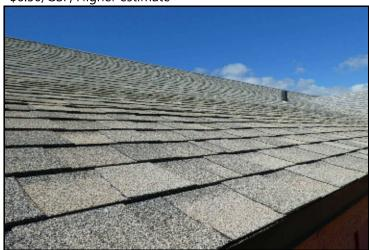
**Evaluation:** Composition shingle roof was installed 11/2003. Good workmanship noted, drip edging and woven valleys. Fair condition and aging normally.
